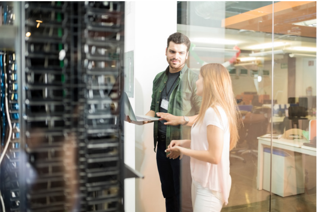
Modern data centre infrastructure supporting institutional cloud ecosystems
